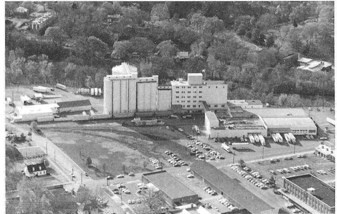
Vibra Screw Bin Activators improved the flow of milled grain products at Southeastern Mills.
