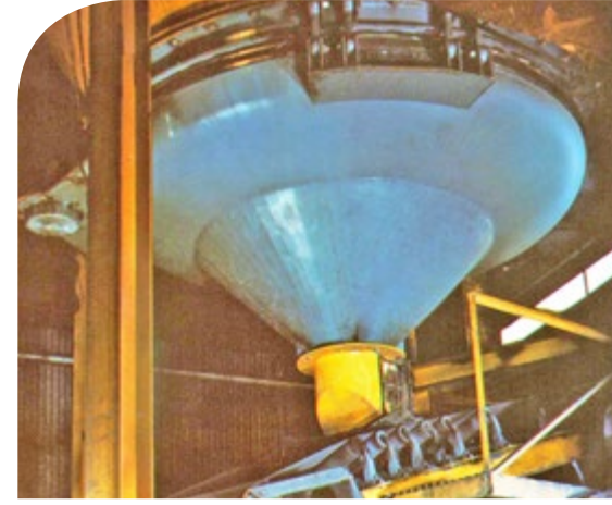
VIBRATED MATERIAL CONTROL NOZZLE MOUNTED on OUTLET
