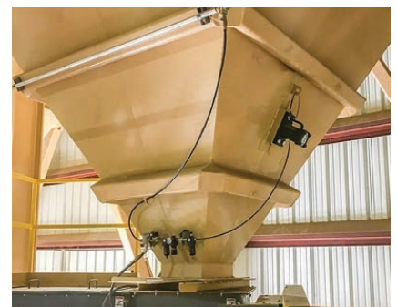
FIGURE 5. Storage-bin vibrators provide a low-cost method to help with material-flow problems, but since they are directly installed onto the bin surface, careful consideration must be taken in their specification
