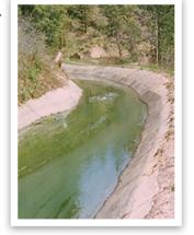
the past a "slug" method was used for dosing. Burlap bags were filled with large copper sulfate crystals and introduced into the feed water. Controlling the concentration was very difficult. If too much copper entered the water it would impart a rusty appearance to the fruit and reduce the value farmers would receive for their crops.
